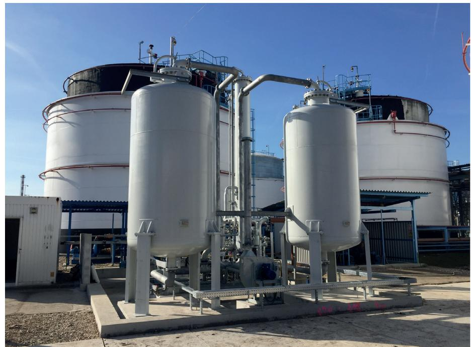
Figure 6 – Vapour recovery unit based on activated carbon and absorption. Cool Sorption, 2019
